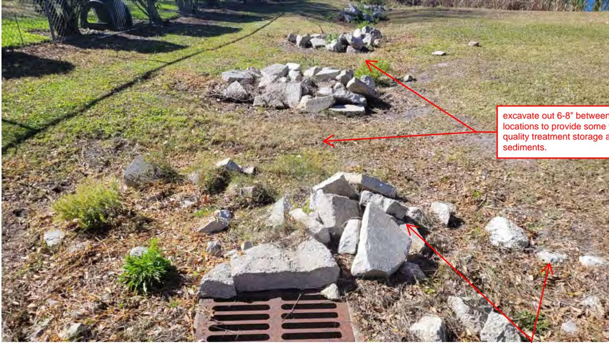
excavate out 6-8" between rip rap locations to provide some water quality treatment storage and trap sediments.
